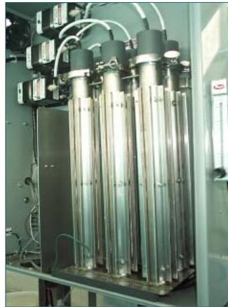
pressurized water, making the tunnel washer at NMMC the first hospital tunnel washer with a pressurized, dissolved ozone system in the U.S. After some initial tuning and balancing of the system to accommodate the continued use of reduced amounts of oxygen bleach, the ozone system has been operating flawlessly.
