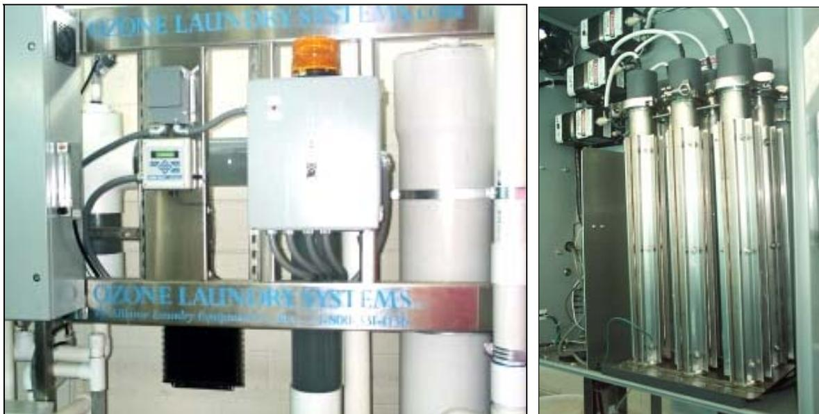
**Figure 3-2 Alliance/IndustrOzone Ozone System (l) and Corona Discharge Tubes (r)**
