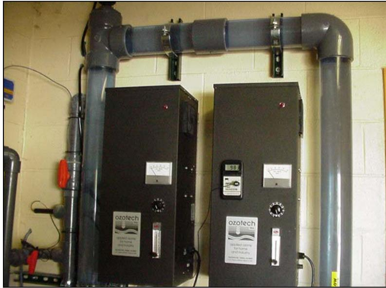
**Figure 4-2 IndustrOzone KA32 Ozone System with Capacity of up to 250 Lbs.**
